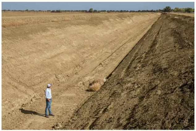
A groundwater recharge basin was built in Huron (Fresno County) to increase underground water storage. Last year, managed recharge of aquifers helped boost California's groundwater supplies. Santiago Mejia/The Chronicle
